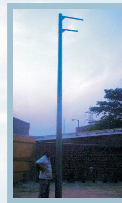
F - Pole Installed at Surat, Gujarat
