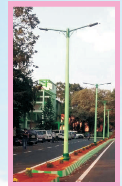
Double Arm Designer Pole Installed at Bhubaneswar, Odisha
