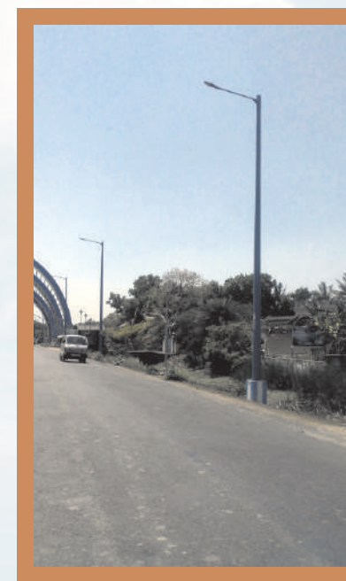
Step Pole Installed at Gateway, Digha, WB
