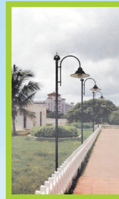
Swan Neck Pole Installed at Surat, Gujarat
