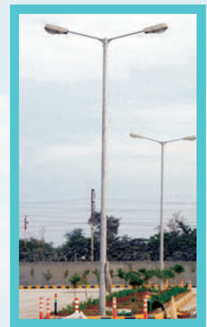
Double Arm Installed at Chennai, TN
