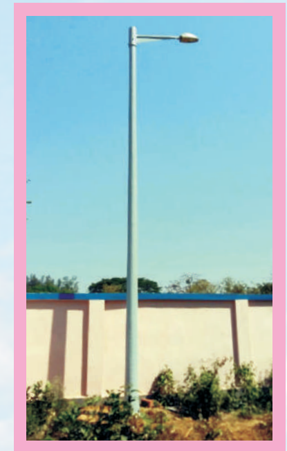
Single Arm Installed at Dankuni, WB
