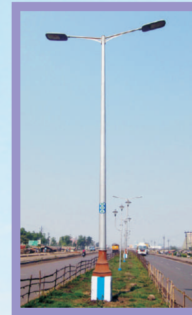
Double Arm Installed at HDA, WB
