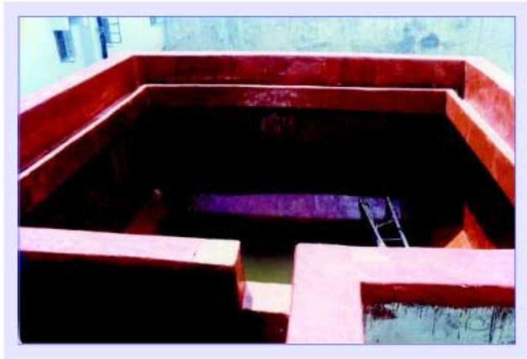
MORTER SCREEDING INSIDE & OUTSIDE OF NATURALIZATION PIT
