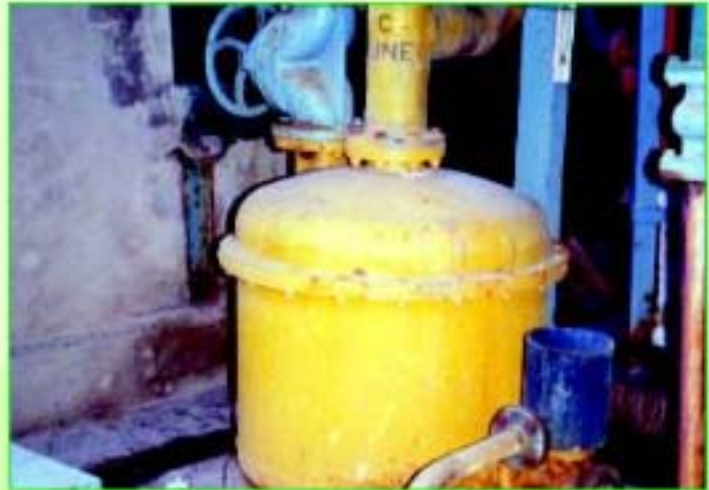
FRP EQUIPMENT WITH PIPING
