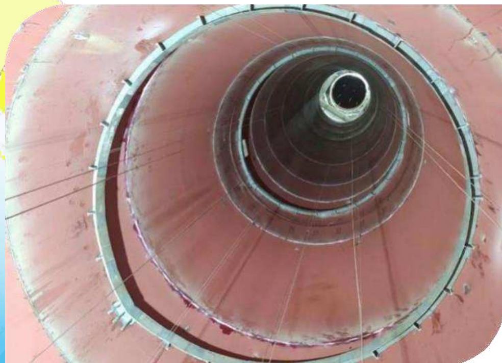
GRP CONDENSATE COLLECTION SYSTEM FOR FGD CHIMNEYS
